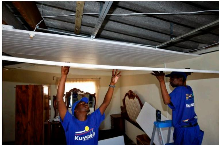
**Figure 9 Insulated ceiling installation**
